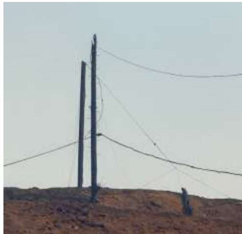
8 9 10 11 12 13 14 15 16 Photograph taken January 8, 2025, showing snapped LADWP H-frame poles 17 above Temescal Water Tank, with powerlines on the ground.
